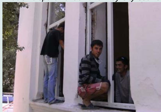
Photo-13: MSU mobilized local communities for reconstructing local schools and kindergartens
