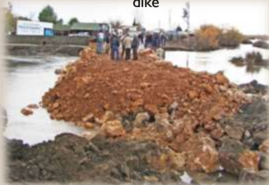
Tale, Pumping station, riconstruction of dike
