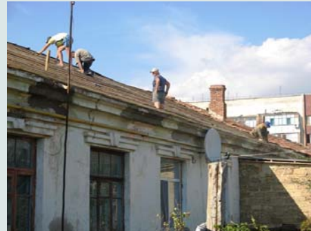
Photo – 9: In progress of roof repairing
