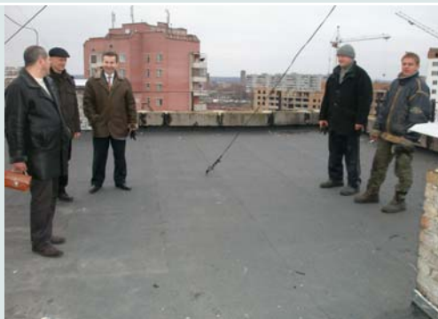
Photo – 12: In process of reconstruction of flat roof at Shukhevycha Street, 2
