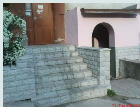
Photo – 14: Repaired entrance halls in the house on 22 Konoval'tsa Street
